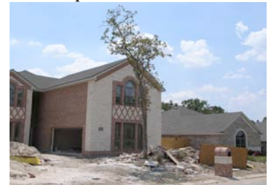
Fig 2. Typical site disruptions during home construction.
