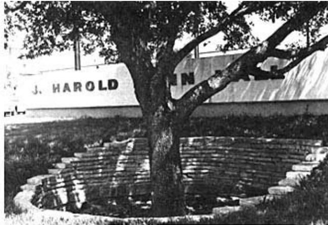
Fig 6. A properly installed tree well and pipe aeration system can protect a valuable landscape tree from damage as a result of fill soil placed over the root system.
