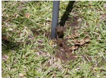
Aerating with water through PVC
